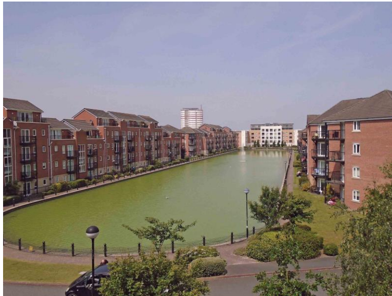
Housing on the site of the former Graving Dock No. 4 of Herculaneum Dock. (Phil Nash, Wikimedia Commons CC BY-SA 4.0 & GFDL)
